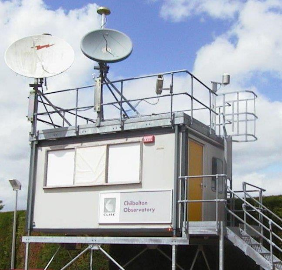
The receive cabin at Sparsholt in Hampshire
