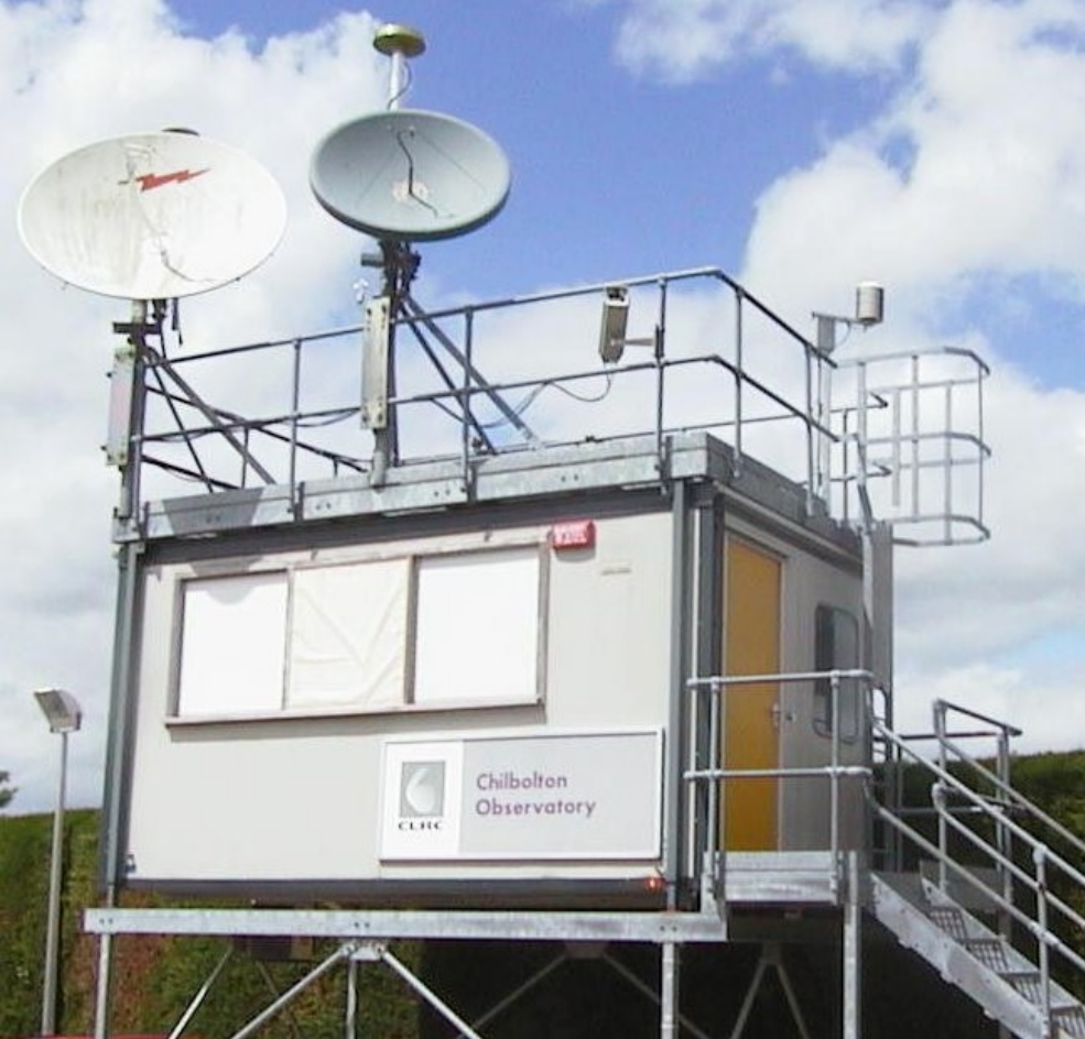
The receive cabin at Sparsholt in Hampshire
